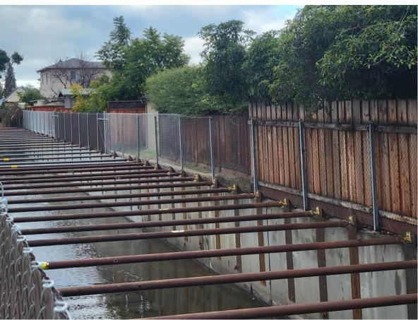
Estudillo Canal Storm Damage - Channel Wall Reconstruction and Temporary Bracing Downstream of Manor Blvd., San Leandro
