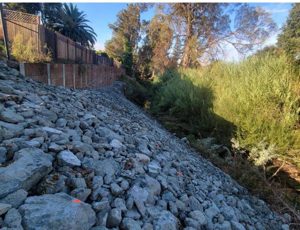
San Lorenzo Creek Storm Damage -Temporary Embankment Stabilization Behind Wingate Way, Hayward
